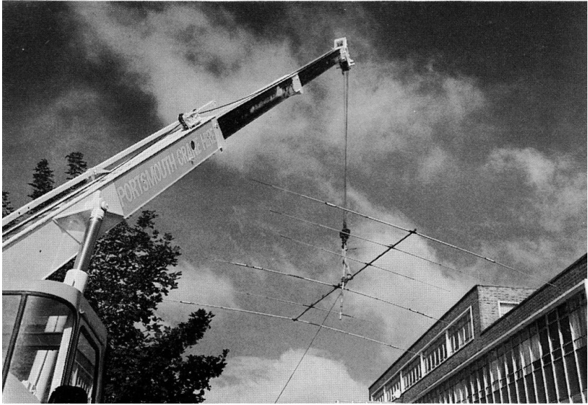
The TH6DXX being removed from the 'new' HQ Shack in the Physical Training and Recreational Building in HMS Mercury
