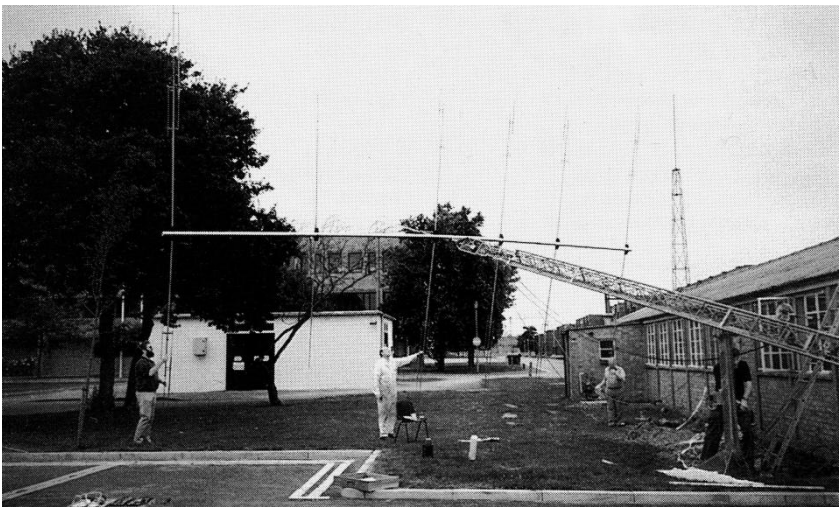
The TH6DXX being fitted to the mast in HMS Collingwood
