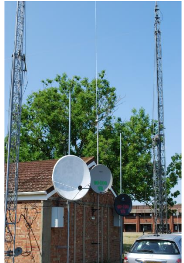
The east end of the HQ Shack showing the satellite dishes and the new multi-band vertical aerial.
