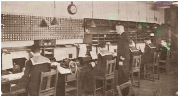
RTT terminal positions for fixed services showing transmitter indicator board
