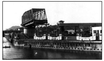
gates while the ship is moving into the lock, a heavy chain is stretched across the lock, well in front of them. Once it is clear that there is no danger, the chain is lowered to the bottom of the lock to let the ship pass. Passage through the locks was a fascinating procedure. The whole process ran like a well-oiled machine.
