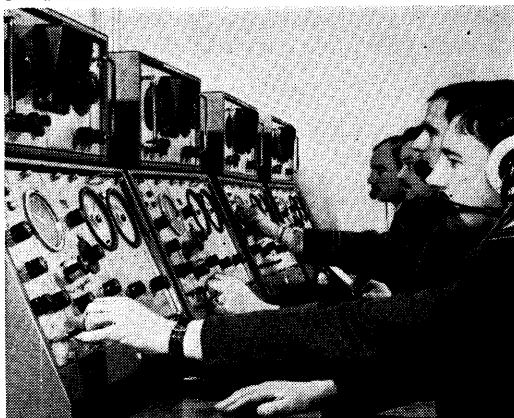
Simulator Target Control Units in Equipment Room, Central Air Traffic Control School, Royal Air Force, Shawbury.
